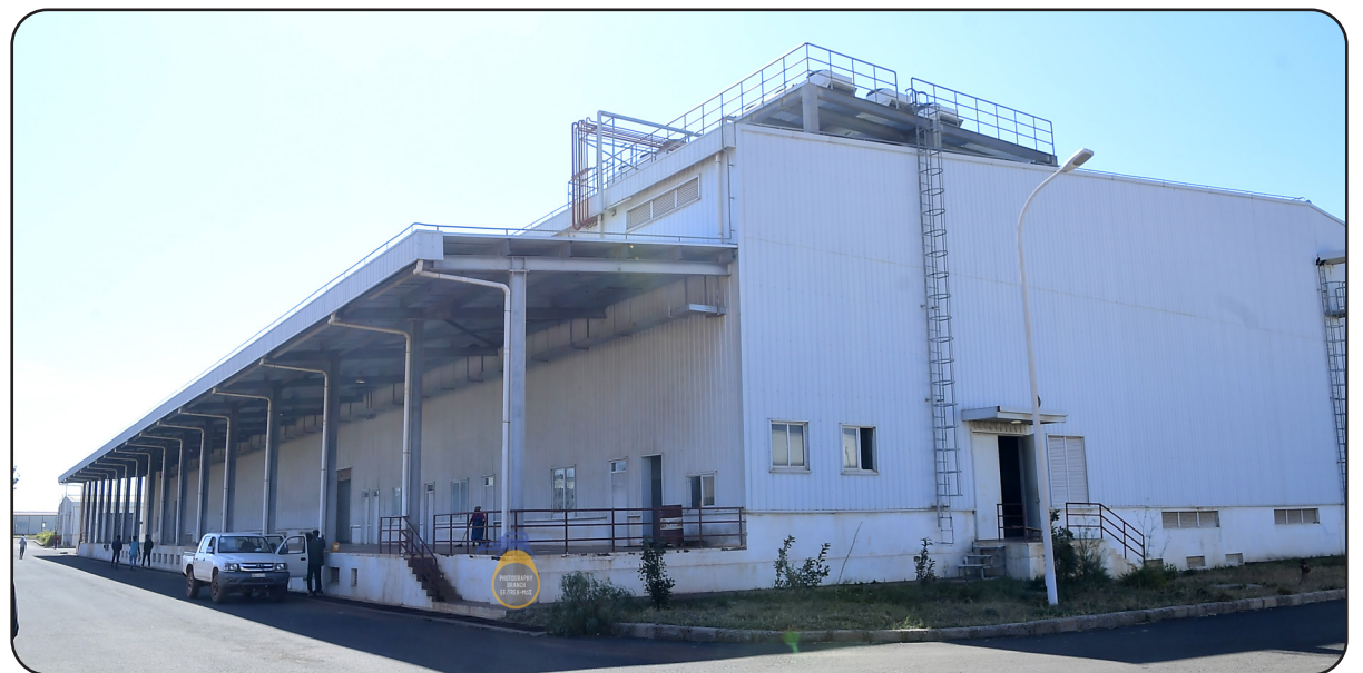
Massawa cooling store
