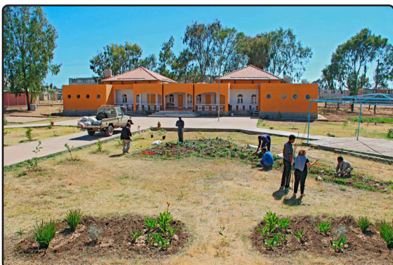
Denden kindergarten inside the Denden Camp
